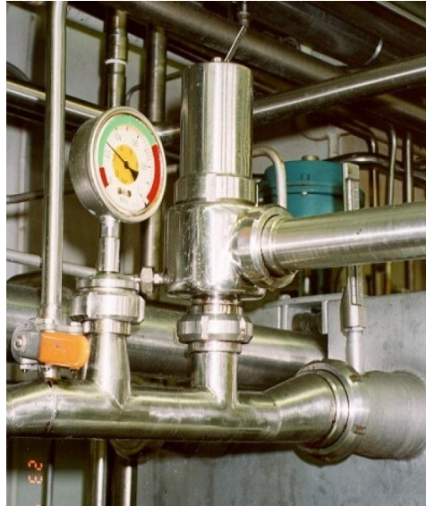
Fig. 42.50 Pressure gauge mounted on a too long tee branch such that unacceptably large dead area is created (courtesy of Huub Lelieveld, personal communication).
