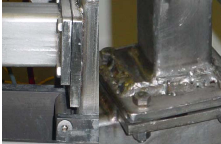
Fig. 42.1 The pits, cracks, crevices, recesses, open seams, gaps, lap seams, bolts and threads will accumulate dirt and will make this equipment uncleanable (courtesy of John Butts, Land O'Frost).
