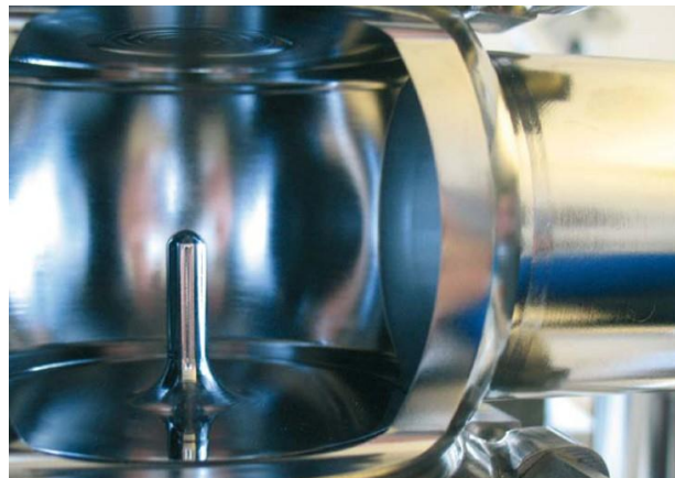
Fig. 42.53 Thermowell integrated into the process, installed by means of a clamp fitting in a standard spherical valve body welded into the piping. The sheath of the probe is welded into one of two blanks which are sealed to the spherical valve body by O-rings fitted into grooves such that there is no metal-to-metal joint on the product side. This way of mounting of a temperature sensor provides a dead-space free, flush transition from the process line to the blank containing the thermowell (courtesy of WIKA).
