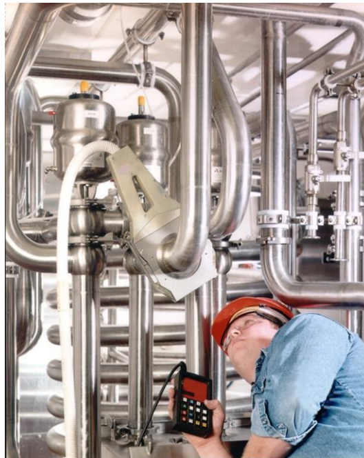
Fig. 42.47 Stainless steel sanitary tubing joints should be made by automatically orbital welding where possible (Kopitzke et al., 2006).
