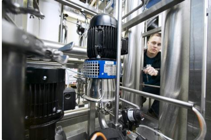
Fig. 42.48 The centrifugal pump is installed in vertical execution, and hence fully drainable through its suction port (courtesy of Hilge).
